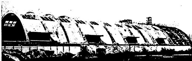
Fig.3 Barrel shell roof in Belgium designed and built by Dyckerhoff and Widmann
