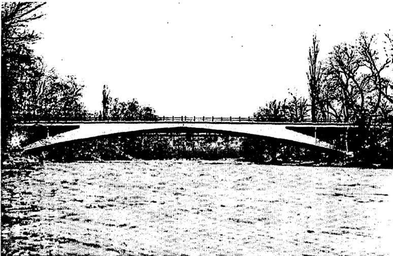
Fig.2 Vessy Bridge profile showing the broken arch and the narrow hinge sections at the abutments and at the crown
