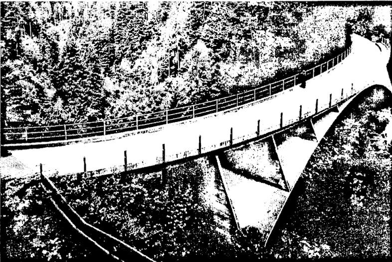
Fig. 5 Schwandbach Bridge with a thin arch integrated to the curved deck by trapazoidal cross walls.
