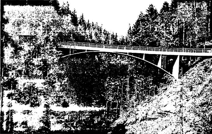
Fig.6 Schwandbach profile showing the thin arch and the stiff horizontal deck
