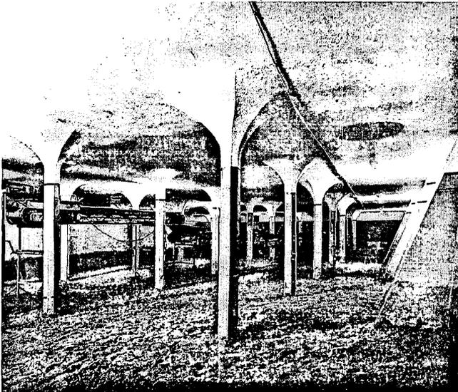
Fig.9 Hyperbolic flared capitals that connect columns to the roof slab of the filter building at Rorschach.
