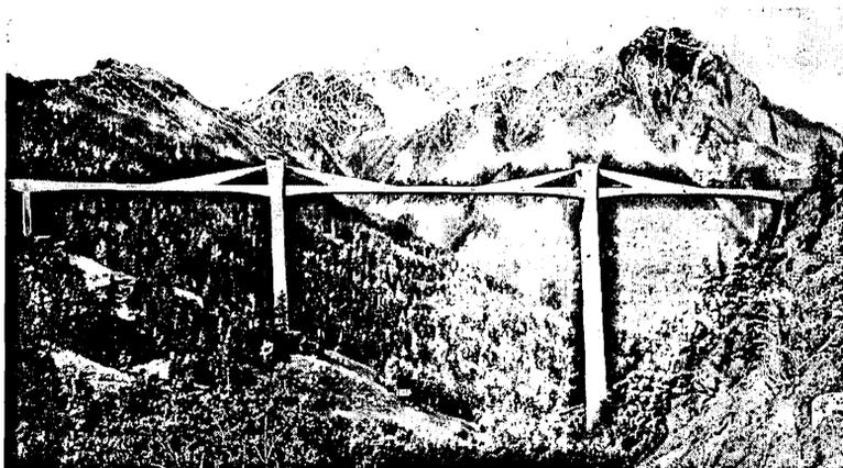
Fig. 18 Ganter Bridge. A low cable-stayed bridge with cables encased in concrete.
