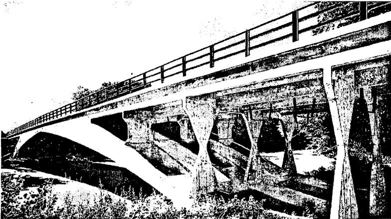
Fig. 4 Vessy Bridge showing the X-shaped crosswalls
