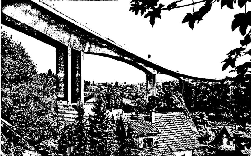
Fig. 17 Felsenau Bridge, prestressed concrete hollow-box cantilever.
