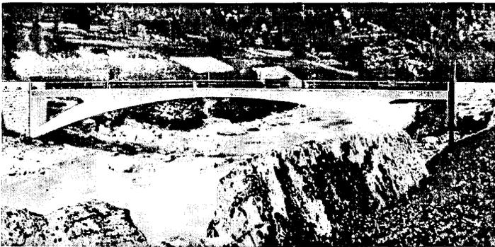
Fig. 14 Tavanasa Bridge showing the profile with the walls near the abutments cut out.
