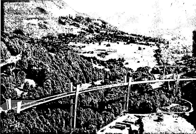
Fig.19 Sunniberg Bridge. A low cable-stayed bridge on slender columns.
