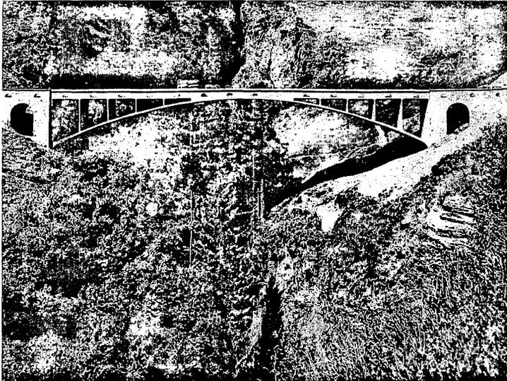
Fig. 7 Valtschielbach Bridge where the parapet stiffens the thin arch.
