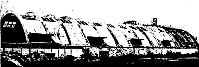
Fig.3 Barrel shell roof in Belgium designed and built by Dyckerhoff and Widmann
