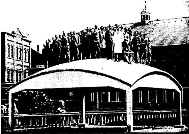
Fig.2 Large-scale model dome designed by Dischinger
