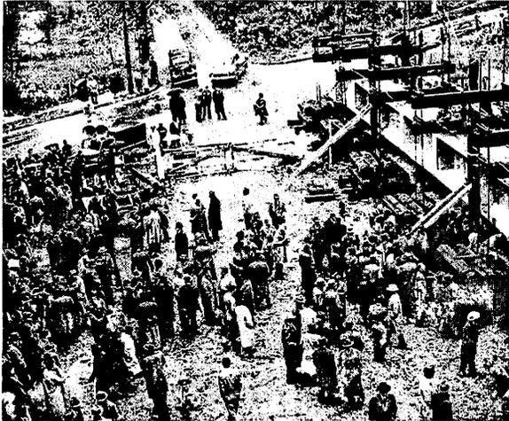
Fig. 13 Test to destruction of one beam at Walnut Lane Bridge.
